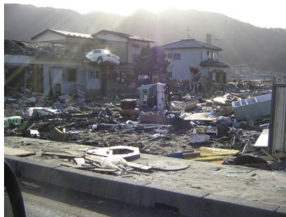
Figure 2. Destruction in Otsuchi.
