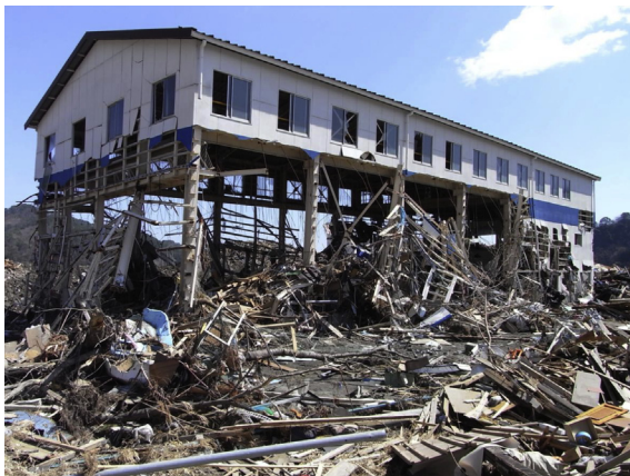
Figure 4. The state of many buildings left standing in Otsuchi.
