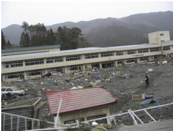
Figure 3. Destruction in Otsuchi.
